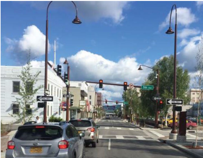
Improvements along Cushman Street
