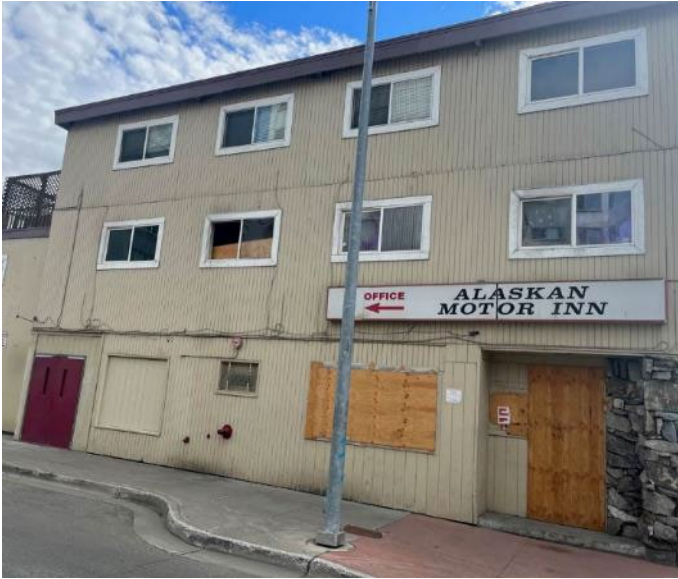
Many vacant buildings need repairs or upgrades.
