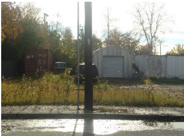
Utility poles placed in the middle of sidewalks make it difficult to walk safely.
